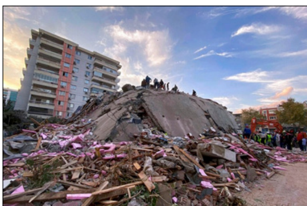
Slika 11: Popolnoma porušena zgradba v Izmirju v Turčiji (vir: https://www.voanews.com/europe/powerful-quake-strikes-major-turkish-city-greek-islands ) Figure 11: A collapsed building in Izmir, Turkey. (Source: https://www.voanews.com/europe/powerful-quake-strikes-major-turkish-city-greek-islands )
