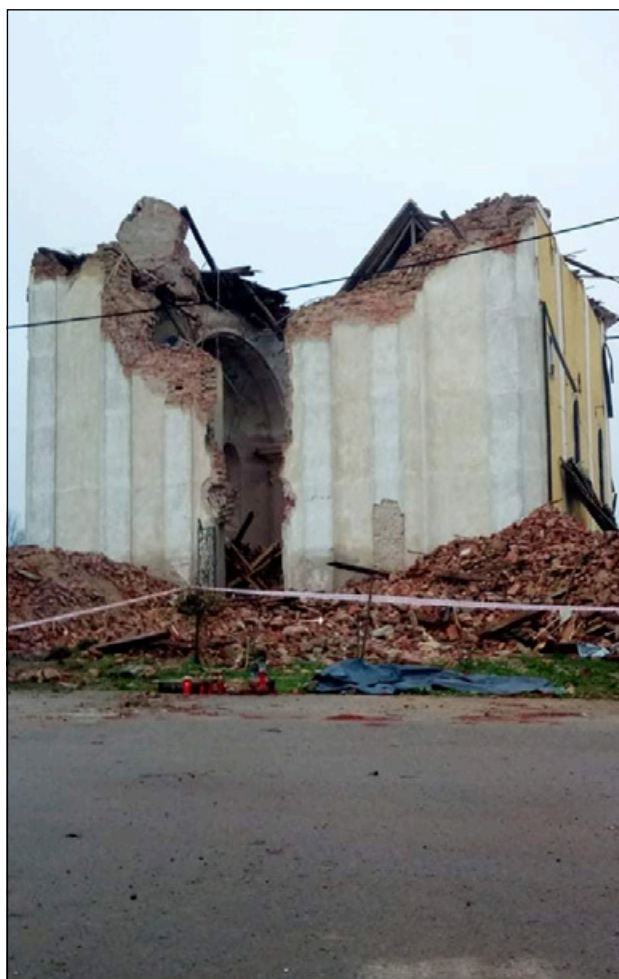
Slika 12: V Petrinjskem potresu (29. 12. 2020) uničena cerkev v Žožini na Hrvaškem (vir: Slavica Gostić, CC BY-SA 4.0, https://commons.wikimedia.org/w/index.php?curid=98597002 ) Figure 12: The church in Žožina destroyed in the 2020 Petrinja earthquake (Source: Slavica Gostić, CC BY-SA 4.0, https://commons.wikimedia.org/w/index.php?curid=98597002 )
