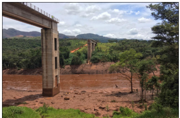
Slika 30: Blatni tok po porušitvi jez v Braziliji konec januarja je tri kilometre dolvodno porušil železniški most (vir: G. Venaglia, commons.wikimedia.org/w/index.php?curid=76197045) Figure 30: After the collapse of a dam in Brazil in late January, a mudslide destroyed a railway bridge 3km downstream (Source: G. Venaglia, commons.wikimedia.org/w/index.php?curid=76197045)
