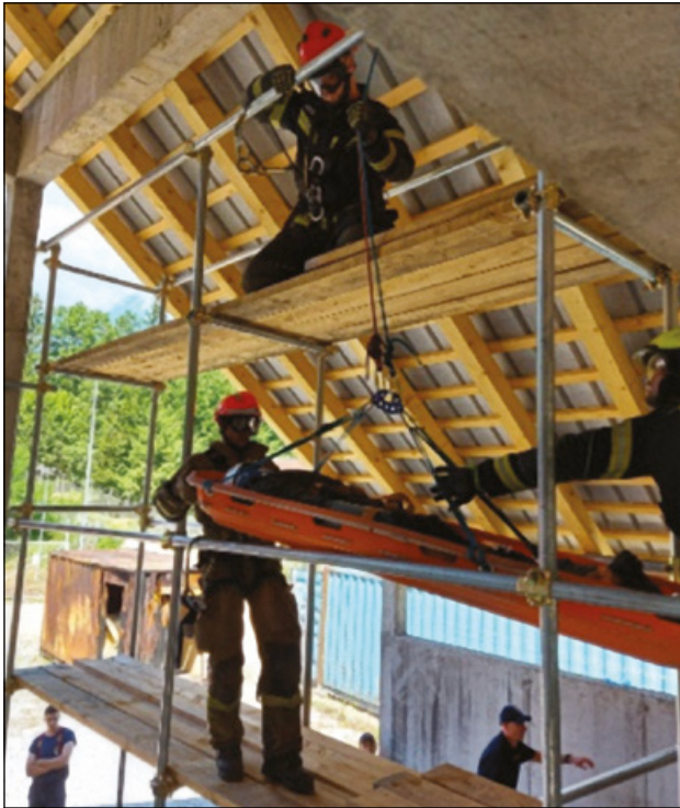
Slika 9: Reševanje poškodovanega delavca na gradbišču (vir: Gasilska šola) Figure 9: Rescue of an injured worker at a construction site (Source: Firefighting School)
