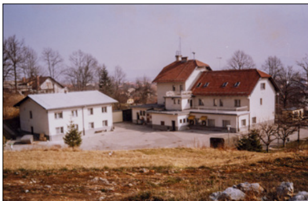
Slika 1: Objekti po prevzemu zemljišča in pred začetkom gradnje (foto: arhiv URSZR) Figure 1: The existing facilities after the takeover of the land and prior the commencement of the construction (Photo: ACPDR archive)
