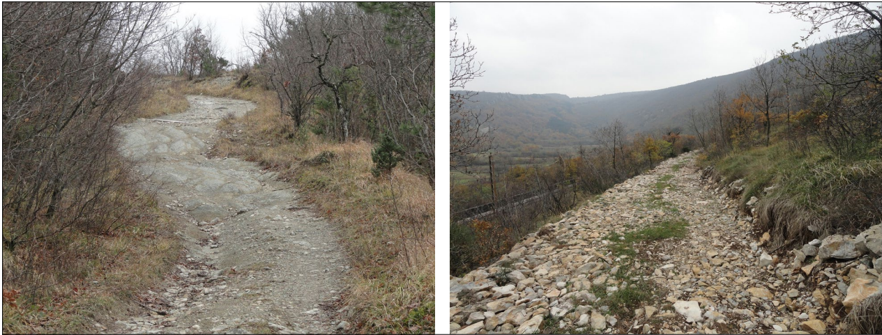
Slika 7: Našo kategorijo 2 odlikuje zadostna širina in izravnan ter delno utrjen planum. (foto: J. Saražin) Figure 7: Our category no. 2 is marked by sufficient width and the flattened out and partially hardened planum (Photo: J. Saražin)
