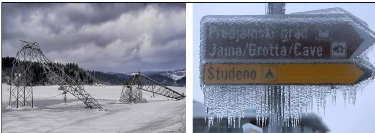
Slika 1: Posledice žleda so bile obsežne. (foto: arhiv URSZR) Figure 1: Sleet caused extensive damage. (photo: URSZR archives)
