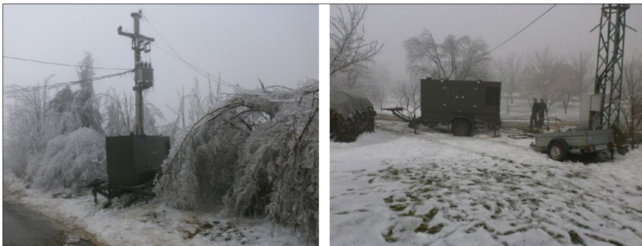
Slika 1: Slovenska vojska v Pivki postavlja agregate (foto: LOGBR) Figure 1: Slovenian Armed Forces installing power generators in Pivka (photo: Logistics Brigade)
