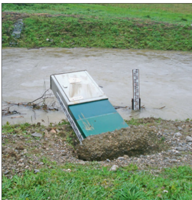
Slika 8: Poplavlni val s 27. na 28. oktober 2012 je porušil vodomerno postajo na Lijaku. (foto: arhiv ARSO) Figure 8: The flood wave from 27 to 28 October 2012 destroyed the gauging station on the Lijak River (Photo: Slovenian Environment Agency - ARSO).
