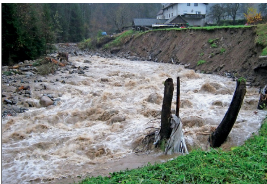
Slika 10: Radoljna pri Radoljni 47 (foto: VGP Drava Ptuj) Figure 10: The Radoljna River at Radoljna 47 (Photo: Water management company Drava VGP Ptuj d.d.).
