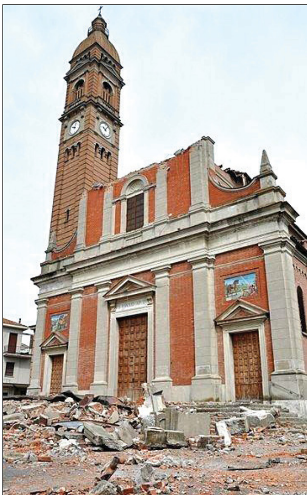
Slika 4: Poškodovana cerkev sv. Pavla v Mirabellu, Ferrara (vir: http://en.wikipedia.org/wiki/File:Chiesa_di_San_Paolo_-_Mirabello_-_Province_of_Ferrara_-_2012_Northern_Italy_earthquake_-_1.jpg )
