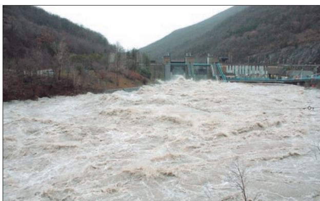
Slika 5: HE Solkan (25. decembra 2009 ob 11.30) (foto: M. Kogoj) Figure 5: The Solkan Hydroelectric Power Plant (25 December 2009 at 11.30 a.m.) (photo: M. Kogoj)
