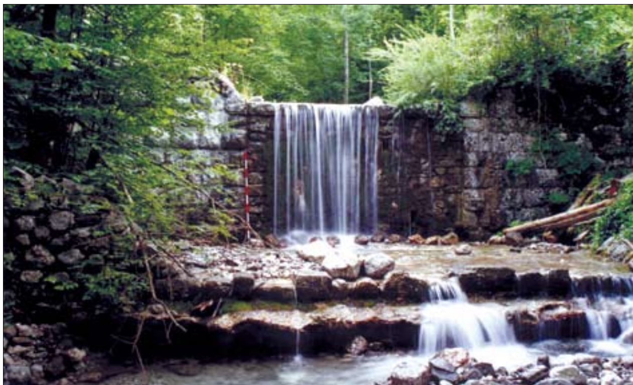
Slika 1. Več kakor sto let stara hudourniška pregrada, zidana v cementni malti (hudournik Šijak) Figure 1. 100-year-old dam in stone masonry (Šijak Flood)
