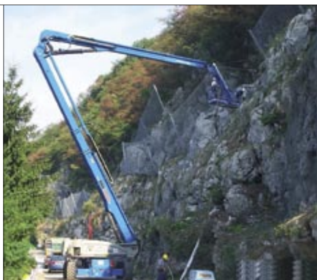
Slika 7 in 8. Izvedba lovilnih podajnih ograj pogosto zahteva uporabo alpinistične opreme (foto: P. Savnik). V bližini prometnic so v veliko pomoč dvižne ploščadi in avtodvigala (foto: A. Rus) Figures 7 and 8. Exacting construction work on the flexible rockfall barrier requires the use of climbing equipment (photo: P. Savnik). Near traffic routes, various kinds of platform and car jacks can be very helpful (photo: A. Rus).
