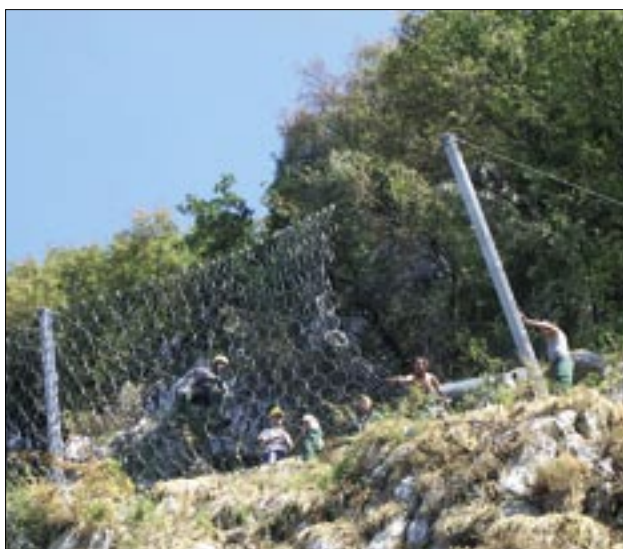
Slika 7 in 8. Izvedba lovilnih podajnih ograj pogosto zahteva uporabo alpinistične opreme (foto: P. Savnik). V bližini prometnic so v veliko pomoč dvižne ploščadi in avtodvigala (foto: A. Rus) Figures 7 and 8. Exacting construction work on the flexible rockfall barrier requires the use of climbing equipment (photo: P. Savnik). Near traffic routes, various kinds of platform and car jacks can be very helpful (photo: A. Rus).
