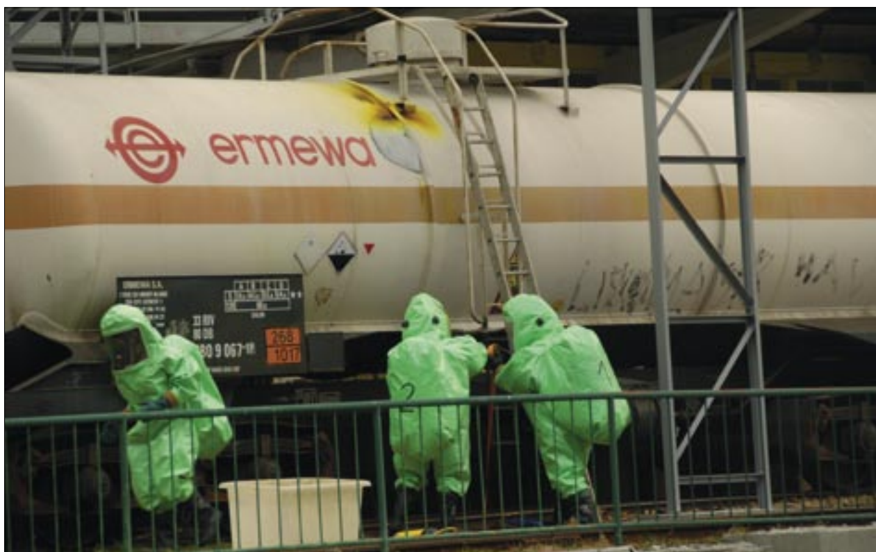
Slika 4. Gasilci iz Gasilskega zavoda Trbovlje so namestili ustrežno objemko na čep in ga tako še dodatno zavarovali. Figure 4. Firefighters from Trbovlje Firefighting Institute fitted the plug with an adequate cap and thus additionally protected it.
