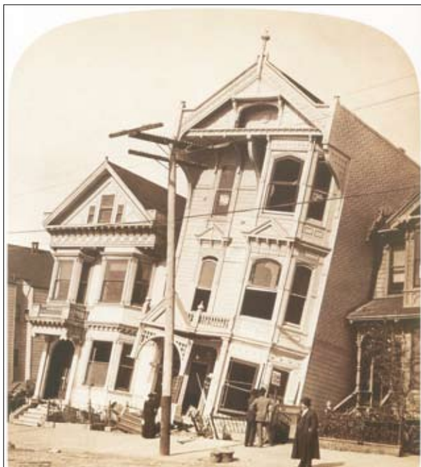
Slika 5. Leseni objekti so se »enostavno« nagnili ali celo podrli, vendar v njih ni bilo veliko žrtev. V njih so bile žrtve le ob požarih. Figure 5. Wooden buildings were simply »expelled« or ruined, but there were not many fatalities in them. There were only deaths in the case of fires.
