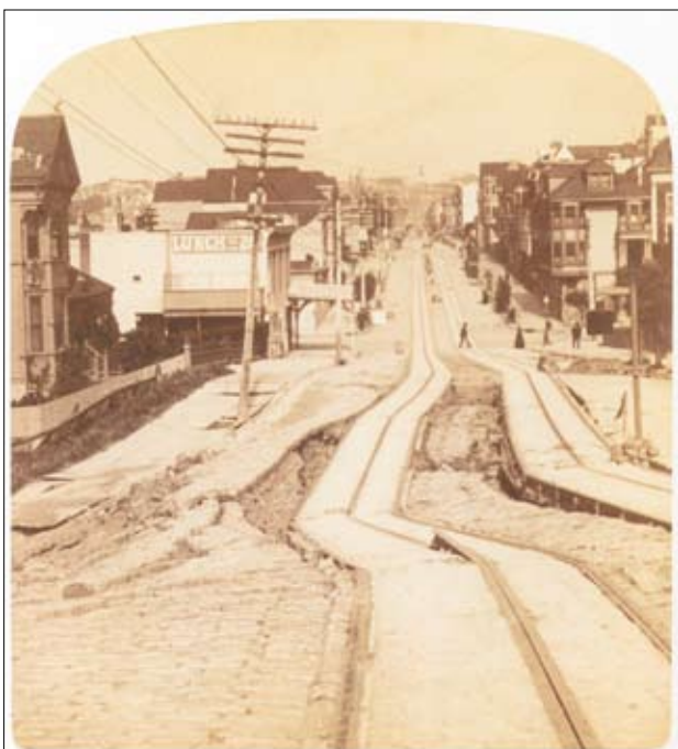
Slika 4. Premiki ob potresu v San Franciscu so ponekod dosegli več metrov. Figure 4. Movements during the San Francisco earthquake in places achieved several metres.
