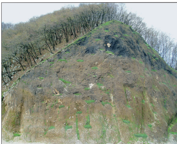
Slika 10. Jesen 2004 – uspešno ozelenjena brežina z vidnimi rastnimi jedri – pogled od spredaj Figure 10. Autumn 2004 – bank successfully made green, with visible plant core – frontal view
