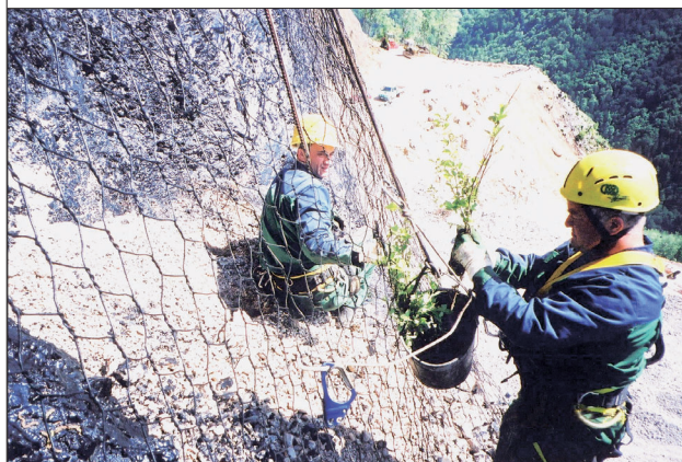
Slika 7. Zasaditvena dela v rastnih jedrih in brežini Figure 7. Planting work in the plant cores and on the banks
