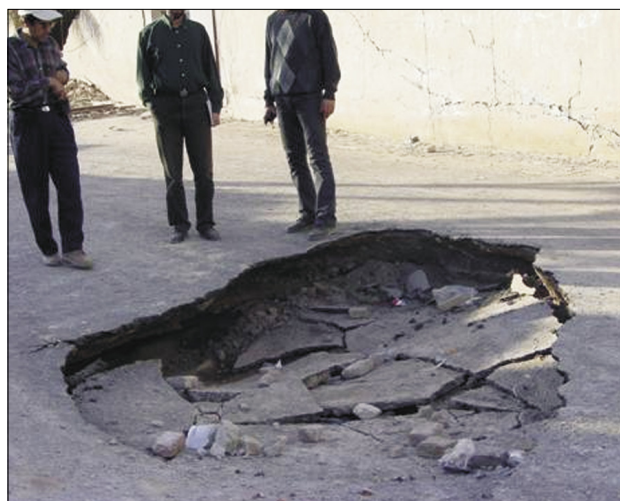
Slika 13. Ponor v bližini glavne ceste v Baravatu; nekateri ponori so nastali pod glavno cesto Figure 13. Sinkhole close to the main road in Baravat; several sinkholes occurred under the main road that has since been repaired
