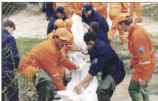
Slika 3. Gradnja nasipa – vodne pregrade (foto: J. Oražem) Figure 3. Constructing embankments as water barriers (photo: J. Oražem)
