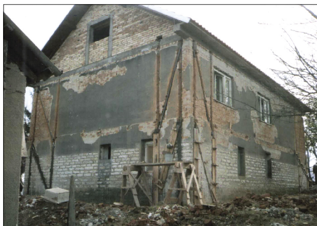
Slika 3. Primer objekta, ki je ojačan s sistemom DC90. Figure 3. A facility where system DC 90 was applied.
