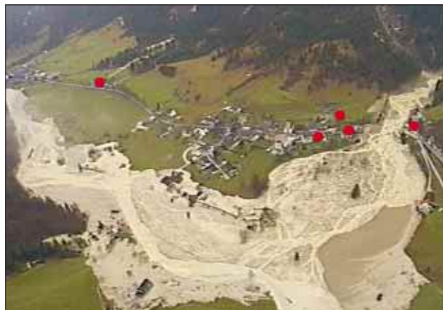
Slika 2. Razporeditev siren mobilnega sistema javnega alarmiranja v Logu pod Mangartom Figure 2. Distribution of sirenes of the mobile public alerting system in Log pod Mangartom
