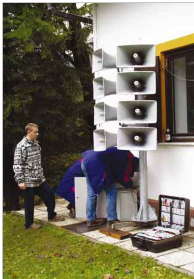
Slika 1. Improvizirana elektronska sirena v Logu pod Mangartom, postavljena dan po nesreči Figure 1. Improvised electronic sirene in Log pod Mangartom, set up one day after the disaster
