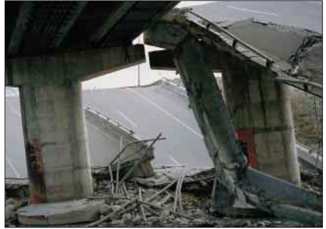
Slika 7. Most porušen v tajvanskem potresu 20. septembra 1999. (foto: R. Vidrih) Figure 7. This bridge collapsed during the Taiwan earthquake on 20 September 1999. (photo: R. Vidrih)
