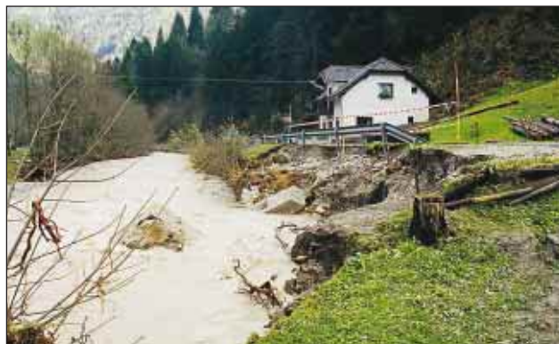
Slika 7. Prometnice ob hudourniških vodotokih morajo imeti ustrezno zavarovane vse odseke, ki so ogroženi ob visoki vodi. (foto: T. Jeršič) Figure 7. Road infrastructure located alongside torrents must have adequate protection for all sections endangered by high water levels (photo: T. Jeršič)
