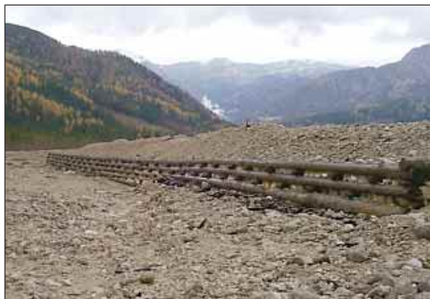
Slika 3. Makekova Kočna – povsem zasuta struga in usedalnik (foto: P. Pejakov) Figure 3. Makekova Kočna – an entirely filled riverbed and sedimentation pool (photo: P. Pejakov)
