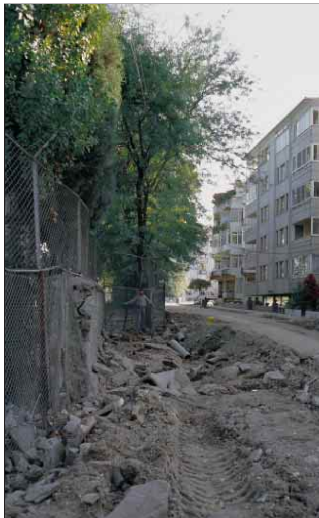
Slika 18. Kamnita ograja se je ob horizontalnem premiku zamaknila za več kot 2 metra. (foto: R. Vidrih) Figure 18. During the horizontal offset, the stone fence was displaced by more than 2 metres. (photo: R. Vidrih)
