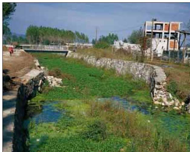
Slika 19. Vsepuvod ob površinskem pretргу so bili objekti zamaknjeni. (foto: R. Vidrih) Figure 19. Buildings were displaced everywhere along the surface of the fault rupture. (photo: R. Vidrih)
