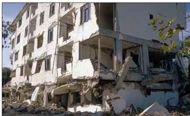
Slika 2. Značilni 6-etažni (2 spodnji etaži sta porušeni) armiranobetonski okvir s polnili (foto: M. Fisching) Figure 2. Typical 6-storey (note that the 2 lower stories have collapsed), reinforced concrete frame with infills (photo: M. Fisching)
