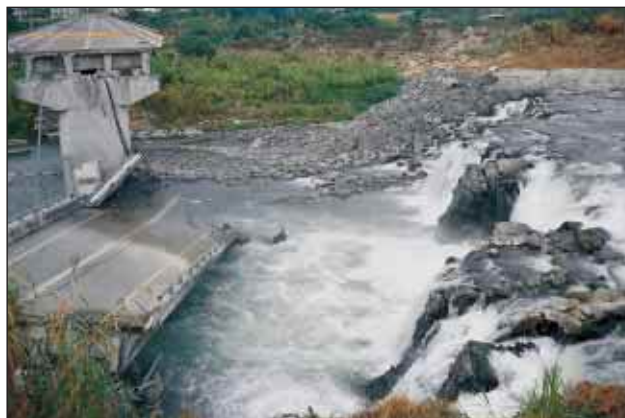
Slika 18. Podrt most na reki Tačja-Hi in ob njem novonastali slap višine okoli 8 m. En blok se je dvignil za okoli 6 m, drugi pa pogreznil za približno 2 m (foto: R. Vidrih) Figure 18. A collapsed bridge on the Tachia-Hi river and a newly-formed waterfall of around 8 m in height. One rock block rose by around 6 m, the other sank by around 2 m (photo: R. Vidrih)
