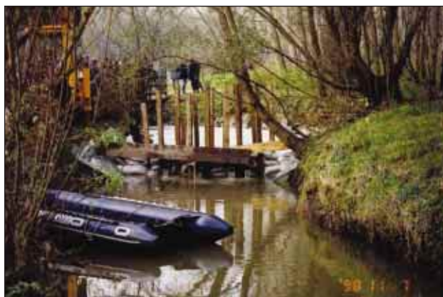
Slika 15. Pripadniki oddelka za tehnično reševanje MO Murska Sobota in VGP Mura so postavili t. i. sifonsko pregrado na rokavu Mure; Ižakovci, 7. 11. 1998 (foto: S. Jauk) Figure 15. Members of the Technical Rescue Department of the Municipality of the City of Murska Sobota and VGP Mura setting up a siphon barrier in a branch of the Mura River (photo: S. Jauk)
