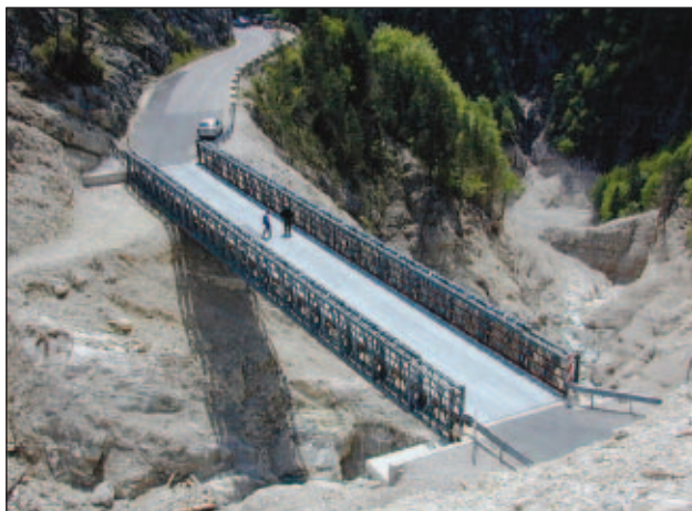
Slika 3. Montažni most čez Mangartski potok pri Mlinču Figure 3. Provisional bridge across the Mangrt stream near Mlinč
