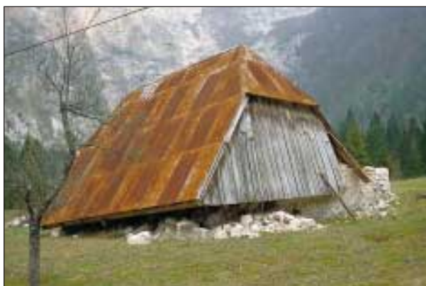
Sliki 15 in 16. Piš je dosegel tudi nekatere zgradbe. Na slikah vidimo, kako je potresni sunek dvignil lopo, ki jo je poznejši piš dobesedno premaknil za več metrov. (foto: R. Vidrih) Figures 15 and 16. Air shocks also reached some buildings. The figures show how the earthquake shock raised a shed, which was later swept several metres away by a subsequent air shock. (photo: R. Vidrih)
