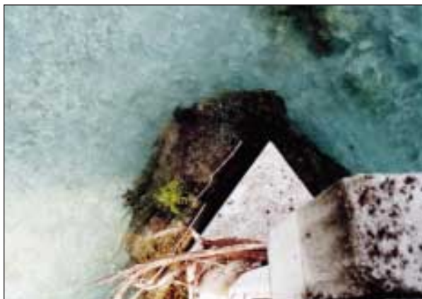
Slika 12. Spodjeden betoniran »kameni zamet« na gorvodni strani poseđenega podpornika (foto: S. Trček) Figure 12. The base of a concreted "stone barrier" on the upstream side of a sunken support has been washed away. (photo: S. Trček)
