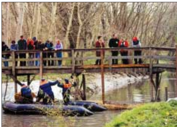
Slika 10. Pripadniki regijskega oddelka za tehnično reševanje so ob pomoči gasilcev preprečili širjenje nevarne snovi po rokavu Mure s t. i. pregrado iz bal slame. (foto: S. Jauk) Figure 10. Members of the Regional Technical Rescue Department, assisted by firefighters, prevented the spread of a hazardous substance in a branch of the Mura River by creating a barrier made of hay bales. (photo: S. Jauk)
