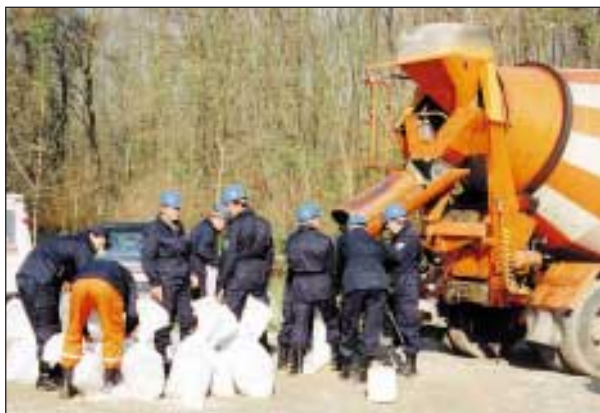
Slika 8. Polnjenje vreč peska z napravo Valostop za postavitev t. i. sifonske pregrade na rokavu Mure (foto: S. Jauk) Figure 8. Filling sand bags with the help of the Valostop device for the purpose of setting up a siphon barrier in a branch of the Mura River (photo: S. Jauk)
