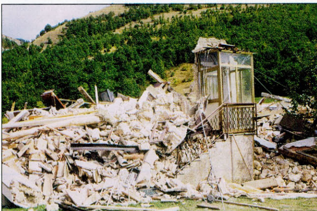
Slika 4. Collecureti, vasica v bližini Colfiorita, je že v prvem potresu utrpela hude poškodbe. Od nekoč velike hiše so ostala cela samo vhodna vrata. Fotografija je bila posneta 3. oktobra 1997. Avtorica te in preostalih fotografij je I. Cecić. Figure 4. Collecureti, a little village near Colfiorita, has already been badly damaged in the first earthquake. Only the doors remain of a once large house. This photo was taken on 3 October 1997. All photos by: I. Cecić.
