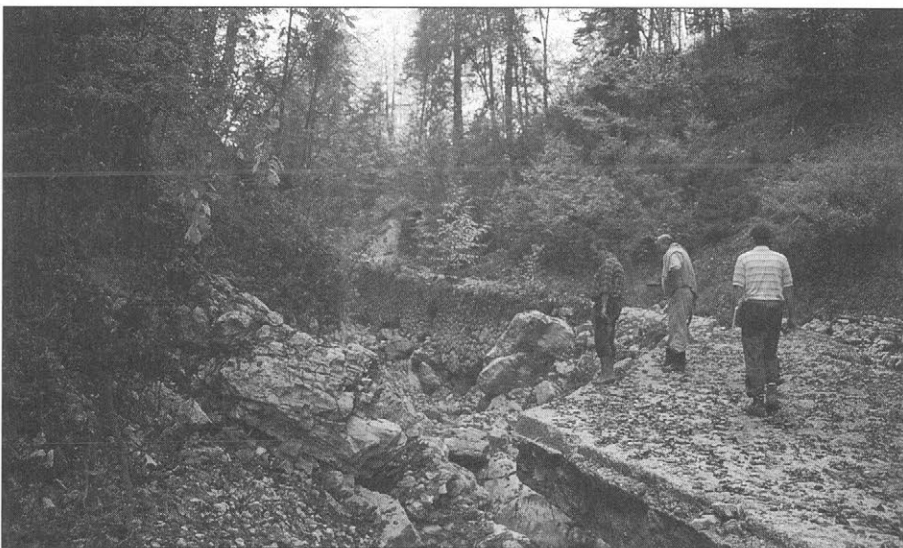
Slika 4. Suhodolnica nad Suhim dolom – odnešena cesta (foto: J. Šeme) Figure 4. The Suhadolnica above Suhi dol – high waters have swept away the bridge (photo: J. Šeme)
