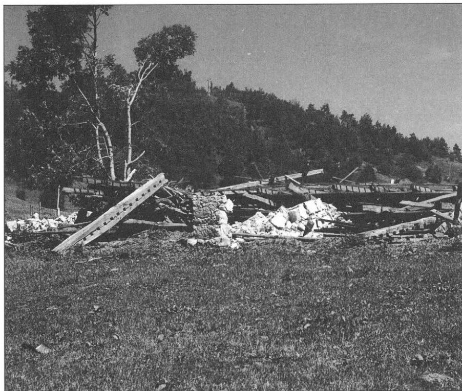
Slika 1. Posledice vetroloma pri Vrhniki 1986 (foto: M. Trontelj) Figure 1. Damage caused by wind, near Vrhnika 1986 (photo: M. Trontelj)
