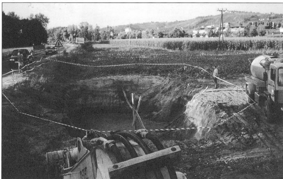
Slika 1. Odkopavanje zemljin in izčrpavanje onesnažene podtalnice (foto: J. Bošnjak) Figure 1. Removal of soil by digging and drainage of dirty underground water (photo: J. Bošnjak)
