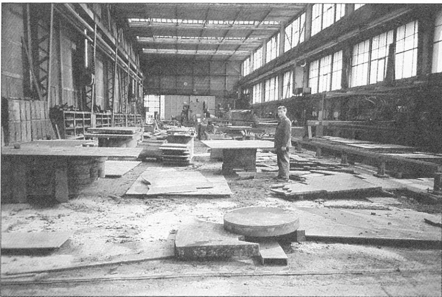
Slika 7. Neurje na območju Trbovelj 28. 6. 1994, blato in voda v eni od večjih proizvodnih dvoran Strojgradnje Figure 7. Vicinity of Trbovlje, June 28, 1994, water and mud damage in one of the larger production facilities of Strojgradnja
