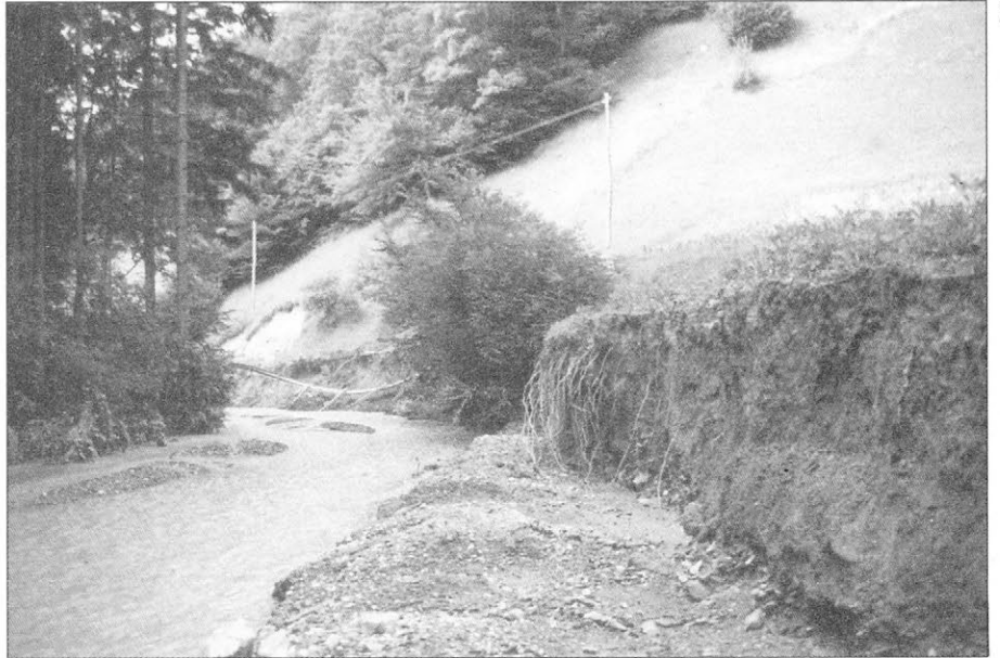
Slika 5. Ozke doline so v večini primerov nastale zaradi erozije vodnega toka; po njih so velikokrat speljane cestne povezave in drugi infrastrukturni objekti, ki zmanjšujejo prvoten potrebni pretočni prerez; v neurjih z večjo povratno dobo ( Q_{100} ali več) si voda z bočno in globinsko erozijo ustvari prvotno stanje; potok Zaplaniščica je na primer porušil cesto skoraj na celotnem izlivnem odseku Figure 5. Roads and other transportation links are usually constructed along narrow river valleys. Because of them, there are many sections of river flow profile that narrower than they would naturally be. During extreme hydrological events (rainfall with 100 or more year return period) the river flow tends to reach its natural state. Side and deep erosion processes cause destruction and destabilisation of many parts of roads, as shown on in the photo of the Zaplaniščica stream on the outflow section
