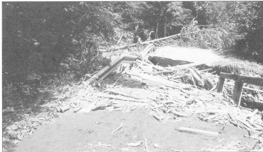
Slika 4. Kotredeščica v Tesni – podrt most na glavni cesti Figure 4. The Kotredeščica in Tesen – devastated bridge on the main road
