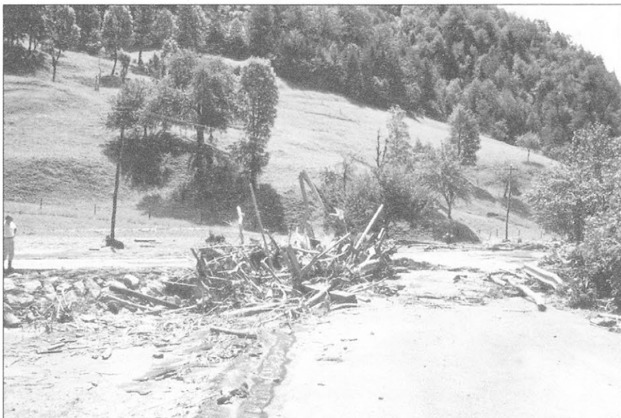
Slika 2. Kotredeščica v Jesenovem – z debli, panji in plavinami zamašena mostna odprtina Figure 2. The Kotredeščica in Jesenovo – bridge clogged with wood and other debris
