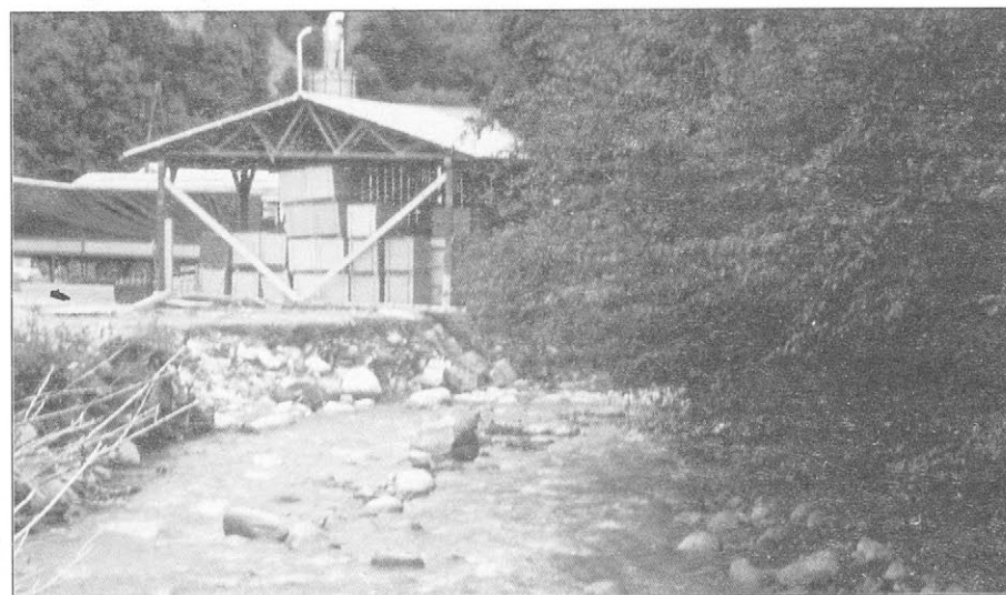
Slika 4. Hudournik Radoljna v Lovrencu: Obrat Marlesa je postavil skladišče kar na neza-varovane brežine Radoljne, ki so jo hudourne vode neusmiljeno spodjedale in odplavljale. Foto: Zoran Fujs Figure 4. Torrential stream Radoljna at Lovrenc: The Marles company erected storage facilities on the unprotected banks of the torrential stream Radoljna while the waters mercilessly flow. Photo: Zoran Fujs
