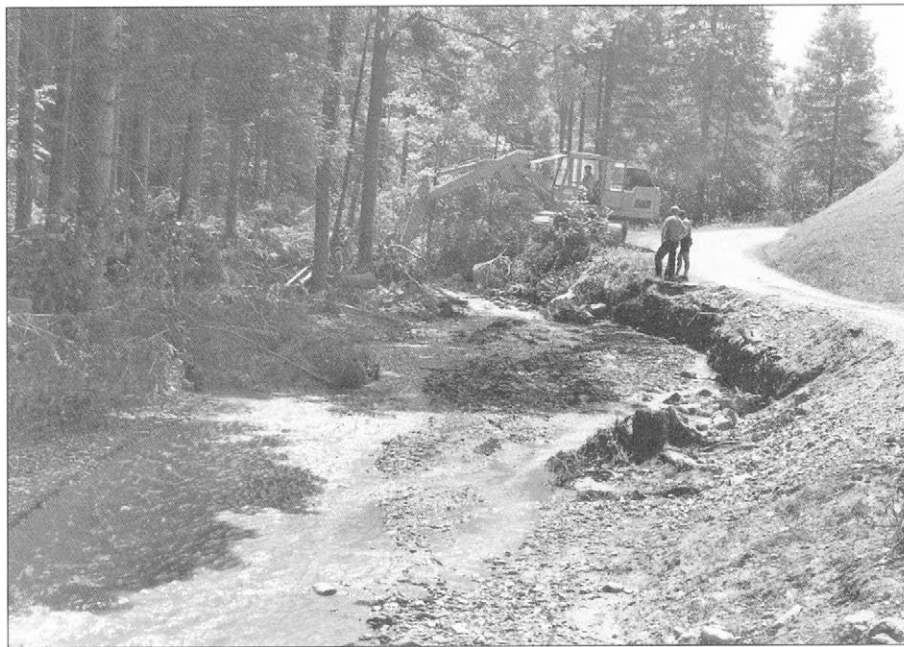
Slika 10. Zaplaninščica tik nad izlivom v Bolsko pri Ločici pri Vranskem: strugo, ki je bila zatrpana s poplavnim nanosom in je ogrožala cesto v Zaplanino, so očistili z bagrom Figure 10. The Zaplaninščica stream above the conjunction with the Bolska river at Ločica near Vransko: the stream bed, clogged with debris, was cleaned
