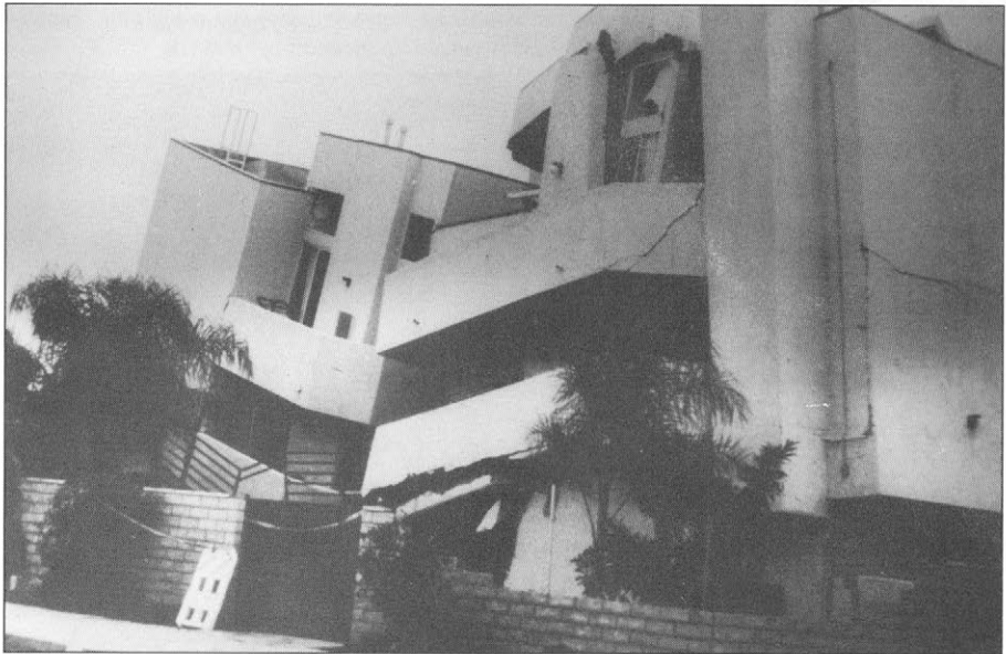
Slika 12. Porušitev večetažne lesene stavbe z mehkim pritličjem. Figure 12. Collapsed wooden multi-story building with a "soft" first storey.
