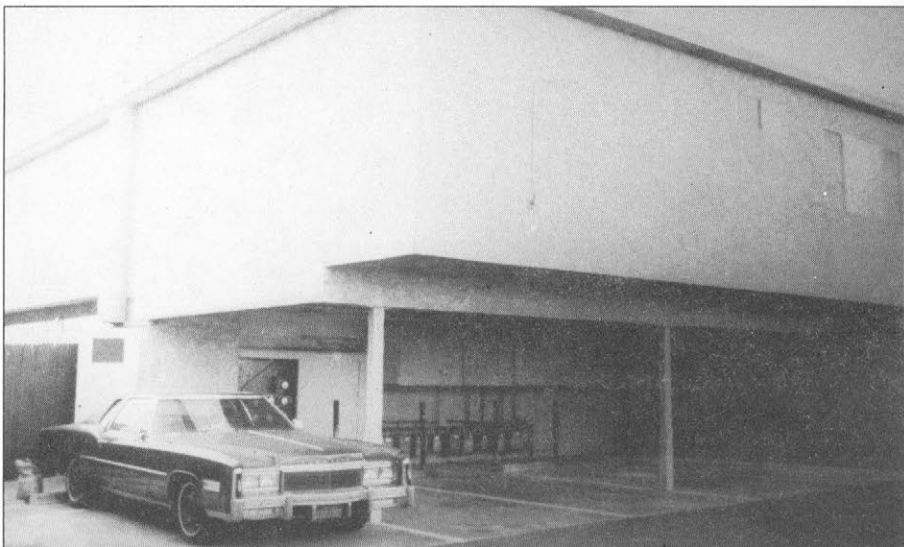
Slika 5. Dvoetažna lesena hiša z "mehko etažo" za garaže (bodite pozorni na plinske napeljavo). Figure 5. Two-storey building with "soft-story" parking (note the natural gas lines).note the natural gas lines).
