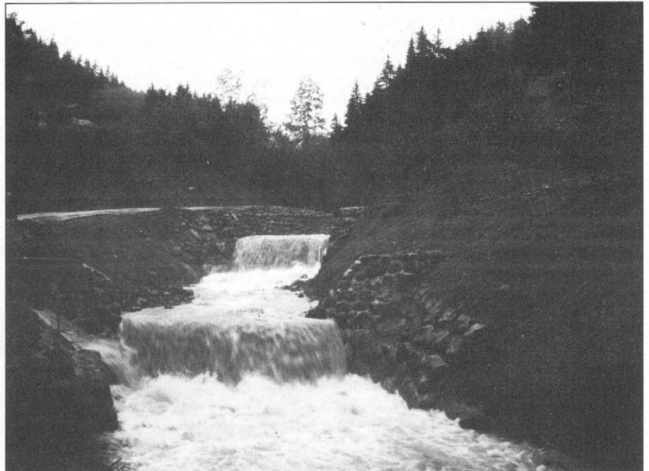
Slika 3. Sistemska ureditev srednjega teka Rogačnika je dobro prestala prvo višjo vodo. (Foto: A. Horvat). Figure 3. The control system in the middle channel at Rogačnik stood up well to the first high water. (Photo: A. Horvat).
